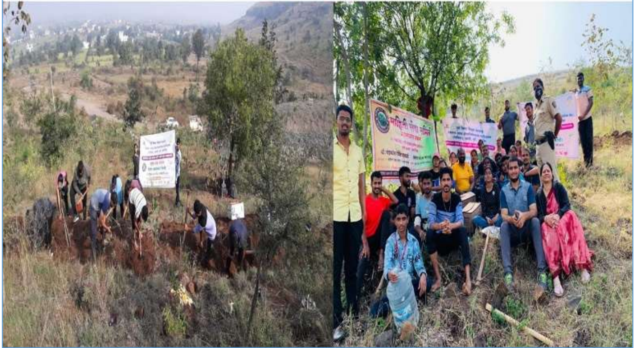
Work for the purpose of water conservation and water horizontally by digging continuous counter trenches(CCT) on the Bakori hills
