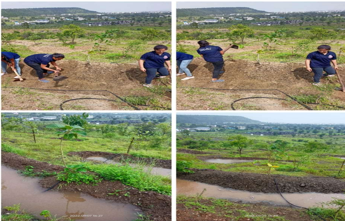
Impact of work done for the purpose of water conservation by digging continuous counter trenches(CCT) on the Bakori hills.
